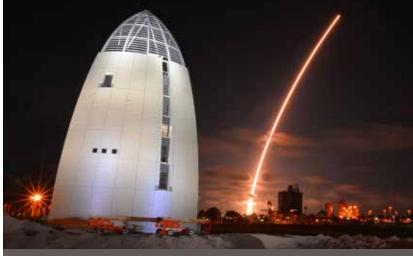
Safety, creativity and attention to detail were top priorities as Kenpat took on the five-month design, prefabrication and installation of 42 concave, tapering structural panelized units and 245 aluminum composite panels for the Port Canaveral
