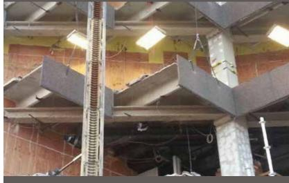
Aggregate Technologies safely removed 340 precast panels weighing more than 2,000 pounds each from a fully operational federal office located on a busy city block by working at night and using two specially designed cranes mounted atop the 22-story building.
