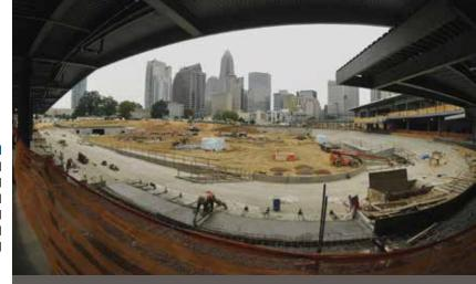
Wayne Brothers completed the turnkey sitework and concrete packages for a LEEDcertified minor league ballpark located in the heart of Charlotte—relying on BIM to resolve issues offsite, coordinate rebar detailing and build custom formwork for the bleachers.
