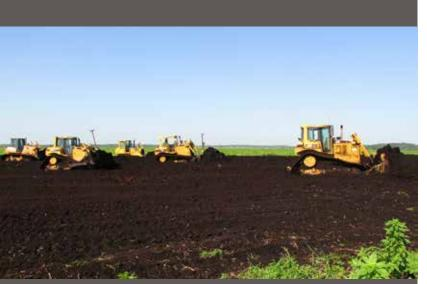
Wondra removed drainage infrastructure, filled seven ditches and installed four spillways—as well as deployed GPS machine control equipment to move more than 24,000 cubic yards of dirt—during the four-month restoration of a 1,600-acre farm.
