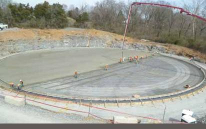
Despite weather delays, multiple subcontractor defaults and having to perform 45-foot-deep excavations adjacent to an operating facility, Brasfield & Gorrie substantially completed this \$13.5 million equalization tank and wastewater pumping station one week ahead of schedule.
